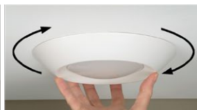
Step 3: Twist and lock into place
