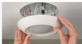
Step 3: Connect the wiring and push
