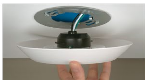
Step 2: Connect the wiring
