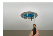
Attach TwistFit Plate to J-box
